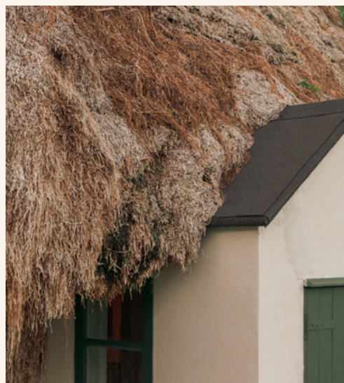
1. Built in the 17th Century, traditional seaweed houses on the Danish island of Læsø represent the first use of eelgrass as a building material.
